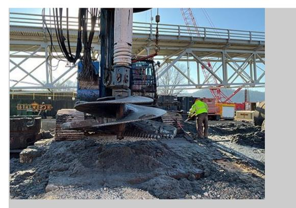
Creating support for the new bridge ... The photo above shows the drill rig and auger used to dig the soil and sand out of a temporary casing by screwing the auger into the material and lifting it out of the hole near the existing Black Hawk Bridge. This process is used to create the shafts that will then be filled with concrete to create the supporting infrastructure of the new bridge at Lansing. Photo courtesy of the Iowa Department of Transportation.
